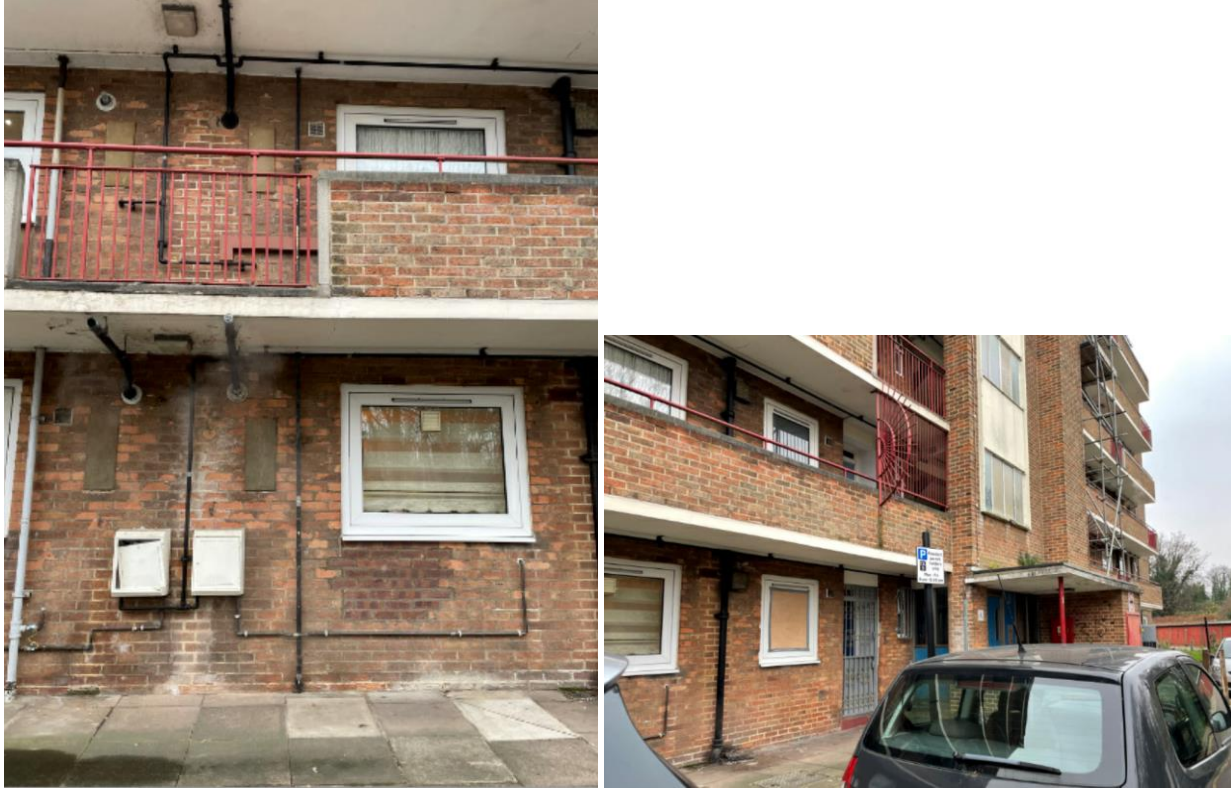
Figures 4 & 5; Nos. 1-24 Remington Road north elevation
